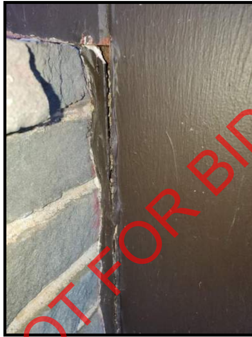
ACM EXTERIOR CAULK AT SIDING (VERTICAL JOINT) AND BRICK, ALSO EXISTS AT WINDOWS AND DOORS
