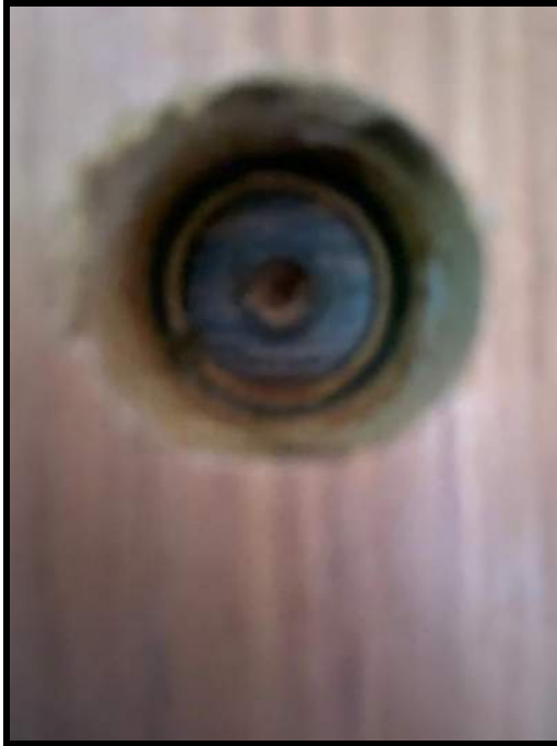
NON-ACM VAPOR BARRIER IDENTIFIED AT FLOOR CORE IN CLOSET
