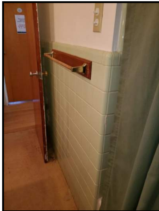
NON-ACM CERAMIC WALL TILE GROUT & THINSET IN BATHROOM
