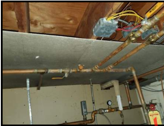
ACM TRANSITE CEILING BOARD OVER FURNACE
