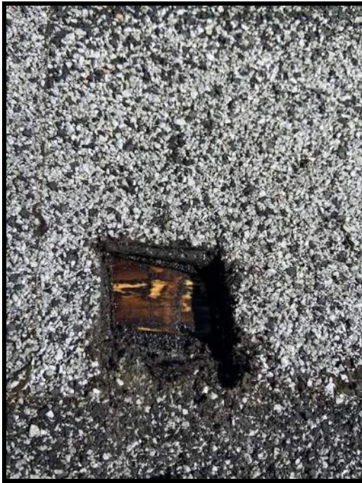
ROOF CORE – SHINGLE AND TAR PAPER ON WOODEN DECK ARE NON-ACM
