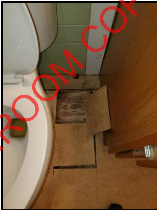
NON-ACM BATHROOM FLOOR TILE AND MASTIC
